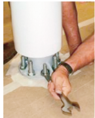
The unit is installed on a floor-mounted pedestal
