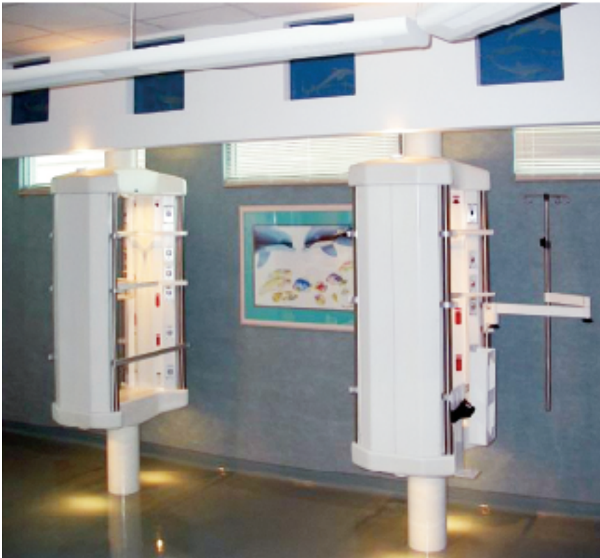
Most bedside equipment and accessories can be contained within the unit's small footprint
