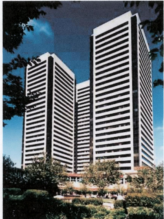
The Sun Life Plaza office towers in Calgary are the site of the first Armstrong ceiling recycling project in Canada. Nearly 250,000 square feet of old tiles were reclaimed.
